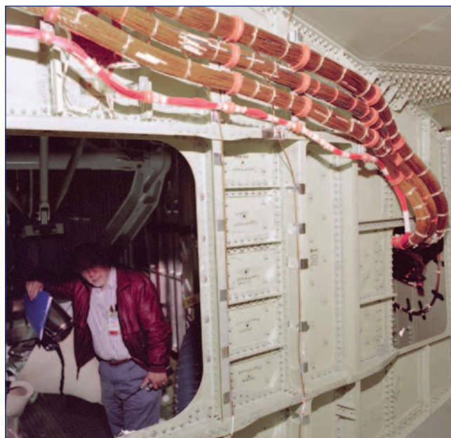
Figure 4.2-3. Typical wiring bundle inside Orbiter wing.
